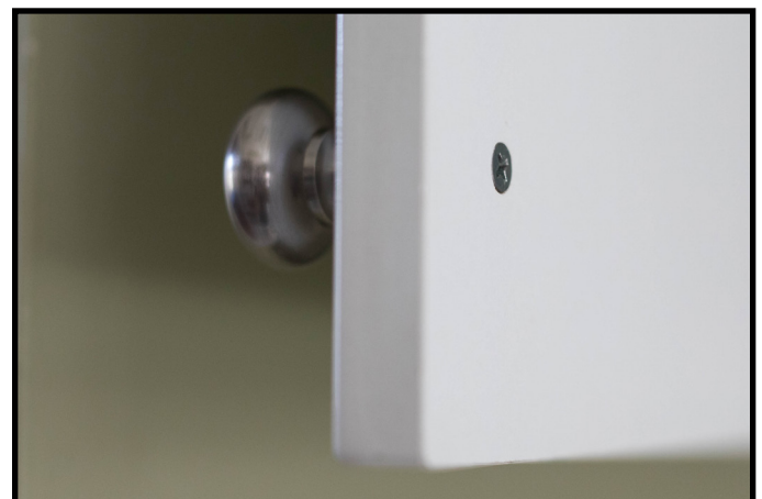
Figure 7.31 - Cabinet Countersink Flush
