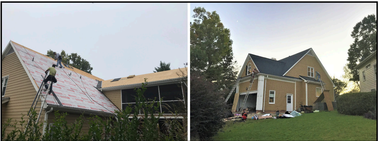
Figure 10.4 - Installing Shingles
