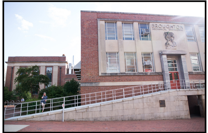
Figure 10.2 - Additional Wheelchair Ramp
