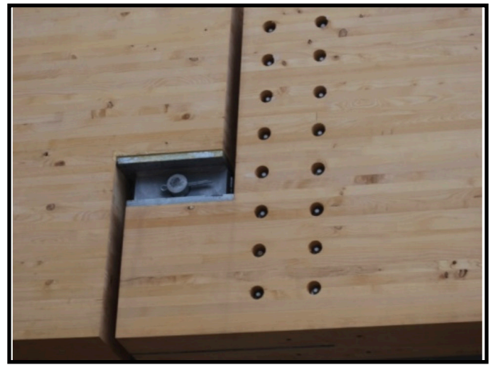
Figure 7.21 - Bridge - Image courtesy of OSHA
